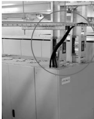
Example of Installation with cable entry from the top
